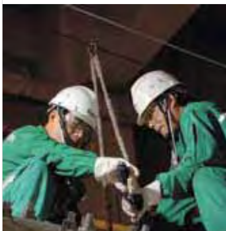
Left: Work at height on raw mill, Chinefarge plant, Beijing, China. Right: Dujiangyan following May 12 2008 earthquake in Sichuan Province, China.
