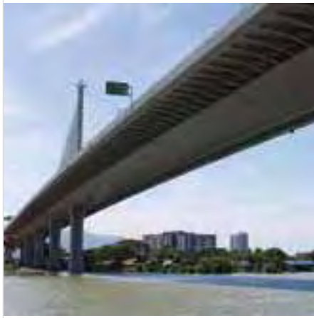
The Sungai Prai Bridge, on the west coast of Malaysia was built using Mascrete™ Pro cement.
